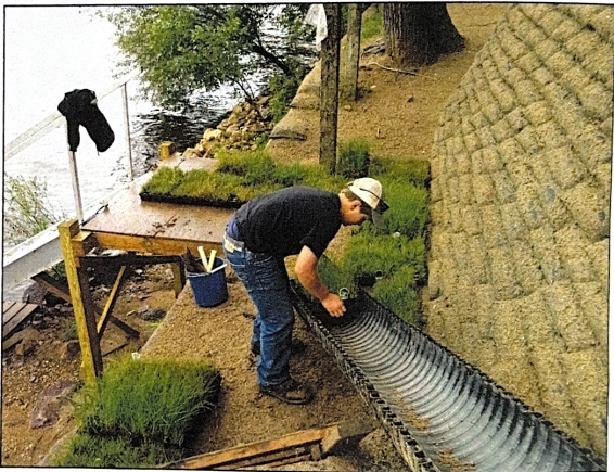
Above: During mid-summer of 2015, installation of steps and removal of timbers were taking place. Below: During early spring of 2014, tube system shown was used to transport native plugs for planting.
