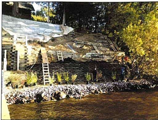
During the fall of 2014, native shrubs were being prepared for planting while soil bag installation was underway.
