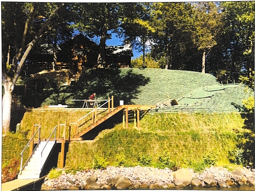
Completed Envirolok progress from the fall of 2015.
