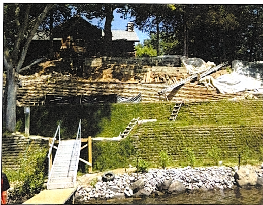
Different stages of the project show the following: vegetated slope on the bottom, constructed wall in the middle, and old existing wall being removed at the top.
